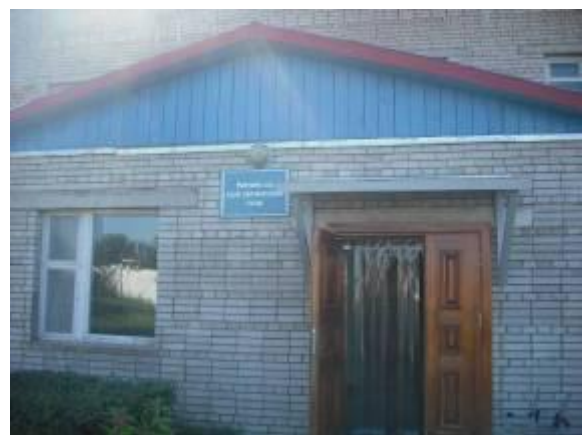
Figure 3.1.2. The office building of Public Utility Service Department
